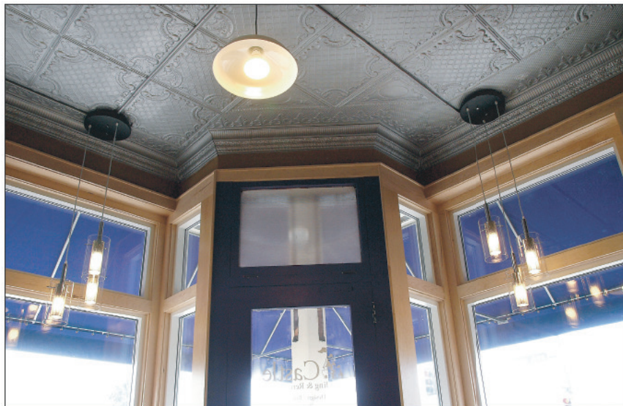
New energy-efficient windows, lighting and a refurbished tin ceiling are featured in this interior view near the main entrance of Castle Building & Remodeling's new Snelling Avenue studio.
